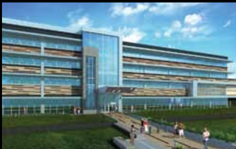
CSRA, Inc. - Bossier City, LA Program Management Services & FFE Installation
